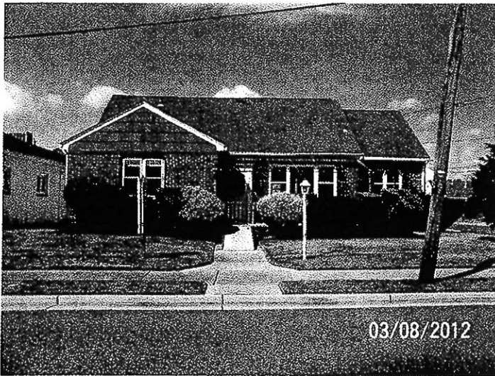
Front View – Date of Photograph: (See Photo Stamp)
